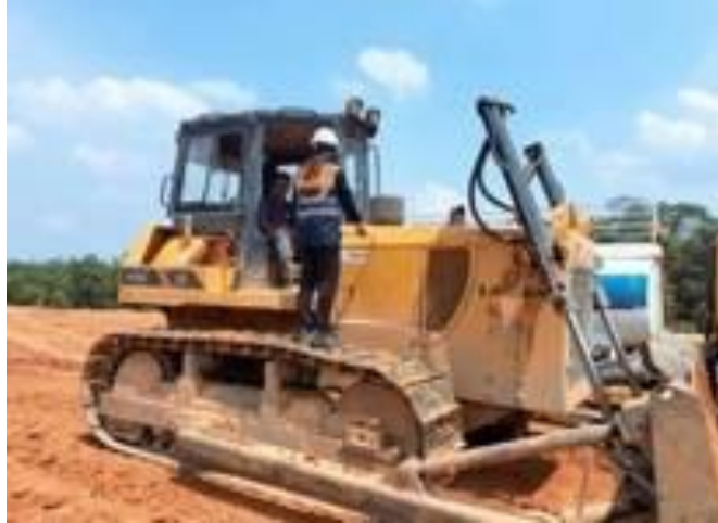
Picture 1. Lifting and Transporting Aircraft in the Riau Toll Road Construction Project
